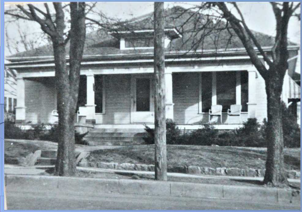
928 W Hickory – Rayzor House Colonial Revival – Built 1912 High Level of Original Integrity
