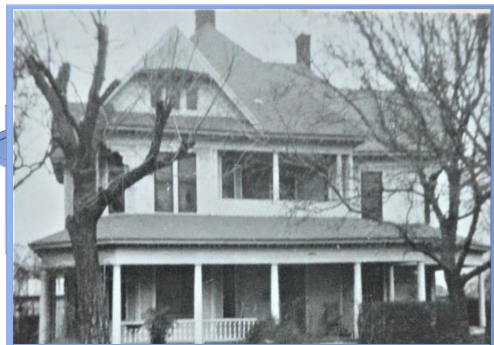
1004 W Oak – Woodward House Queen Anne, Built 1897 High Level of Original Integrity
