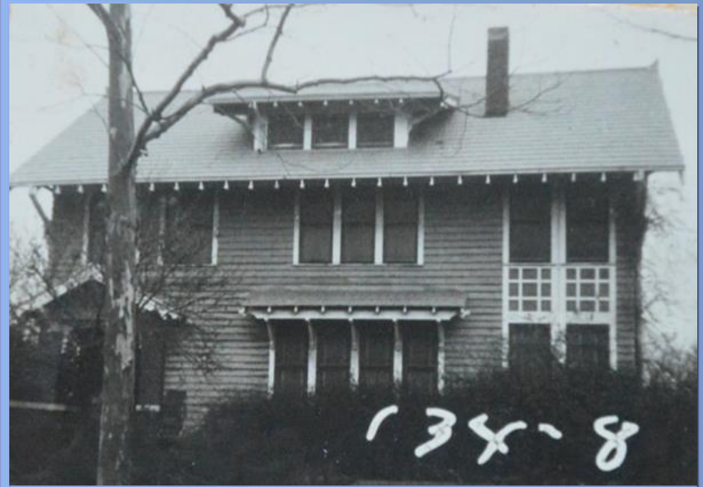
1018 W Oak - Long House Craftsman, Built 1914 High Level of Original Integrity
